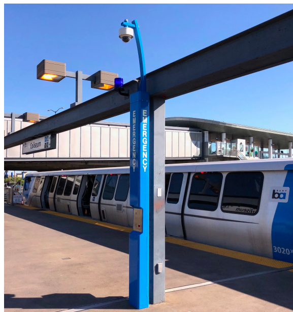
Figure 1: Emergency call box at Coliseum Station (California)
